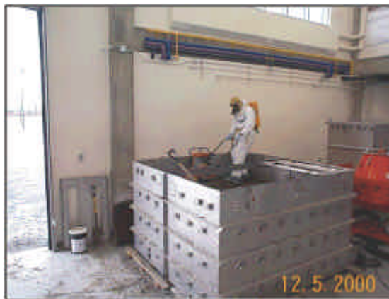
Figure 2. Soil compaction in the tank
