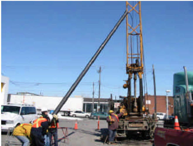
Figure 5. Heating element installation on site.
