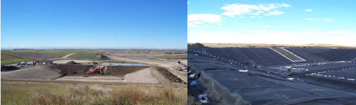
Figure 4. Compacted clay liner and HDPE liner of the cell
