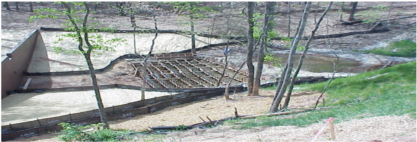
Figure 2 Baffle Grid system designed for 15,000 + GPM, Atlanta, Georgia
