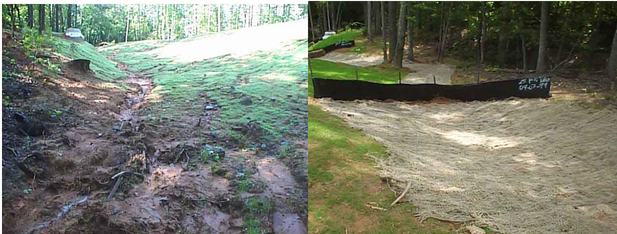
Figure 4 Before and After Soft Armoring application
