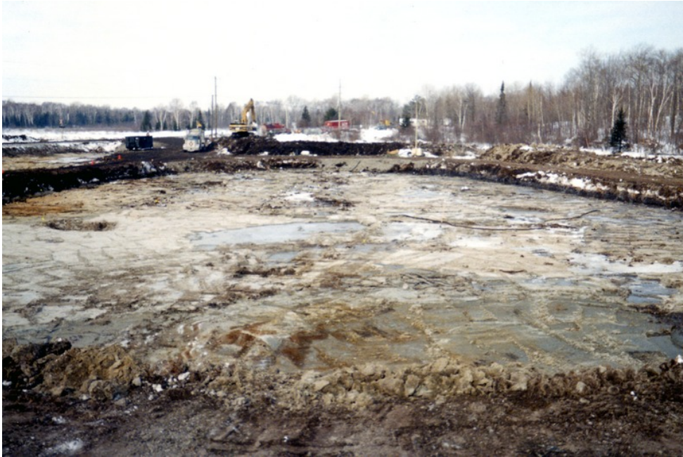
Photograph 1: View of Site at Completion of Initial Remediation Activities
