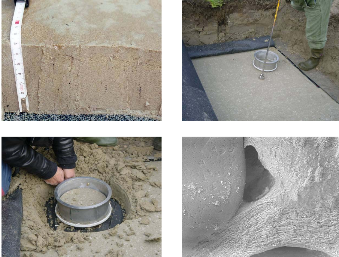
Figure 6 - Pictures of Trisoplast taken during and after excavation
